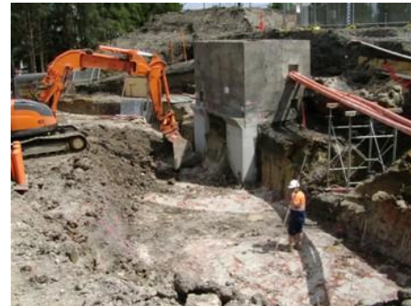
Shoring of existing structures
