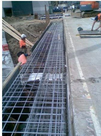
Headstock reinforcing
