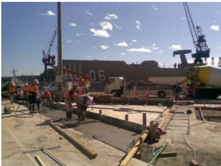
Finishing slab construction
