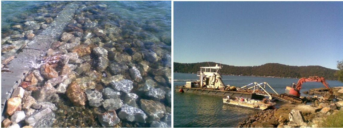
Photograph of Telstra cable protection structure construction
