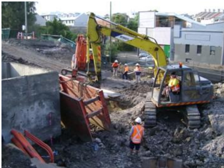
Shoring of existing structures
