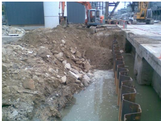
Sheet Pile Caisson
