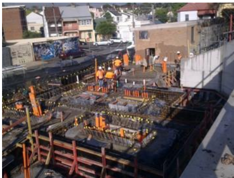
Slab and pit Construction
