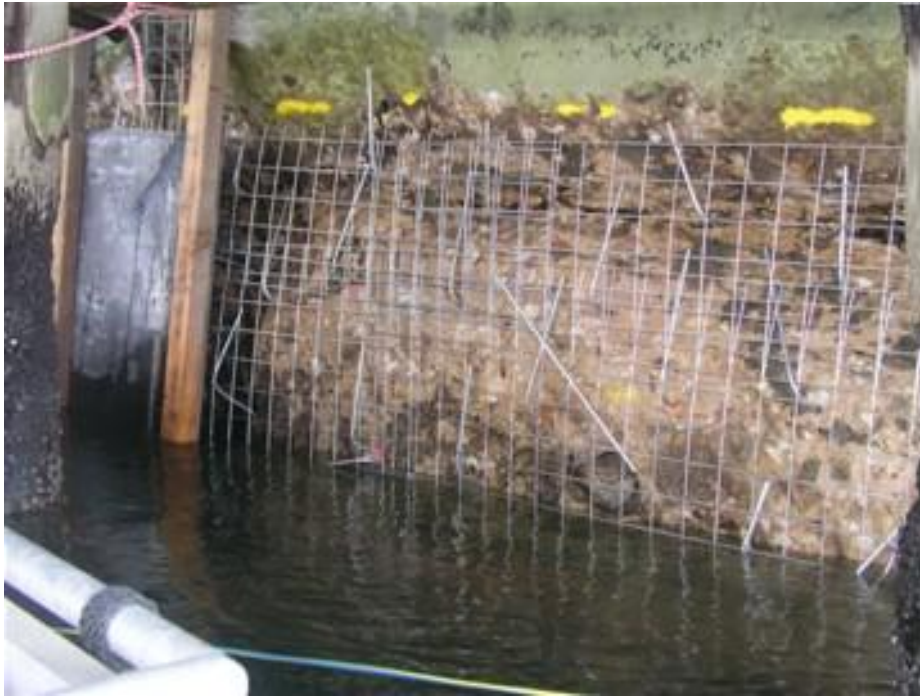
Mass concrete repairs using epoxy dowells and mesh.
