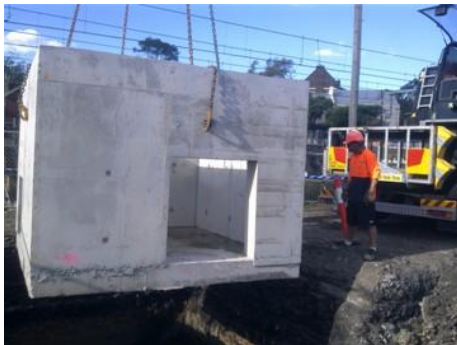
Precast pits used to accelerate program constructed by L&M
