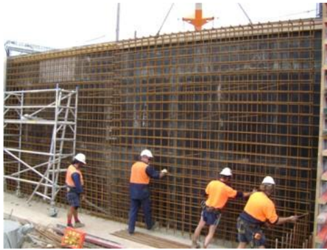
Concrete retaining wall preparation
