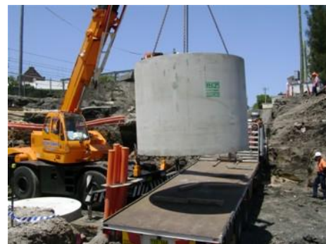
Humeceptor Oil Separator Installation
