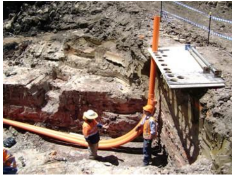
Conduit Templates used to ensure precise positioning of cable routes
