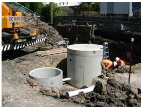
Humeceptor Oil Separator Installation
