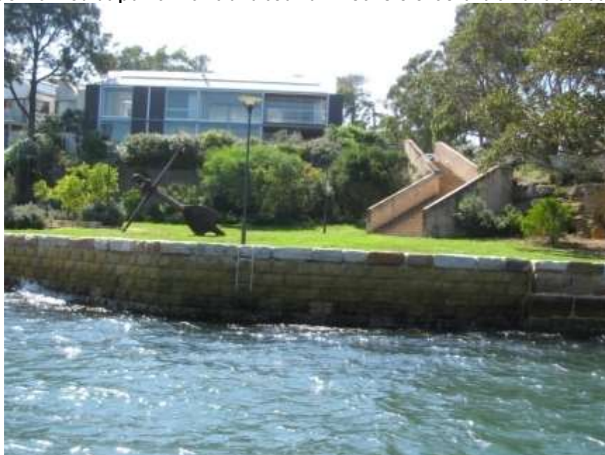
Beach formed as part of works and seawall in concrete loc-a-blok and sandstone
