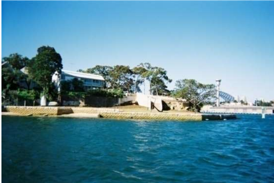
Beach formed as part of works and seawall in concrete loc-a-blok and sandstone
